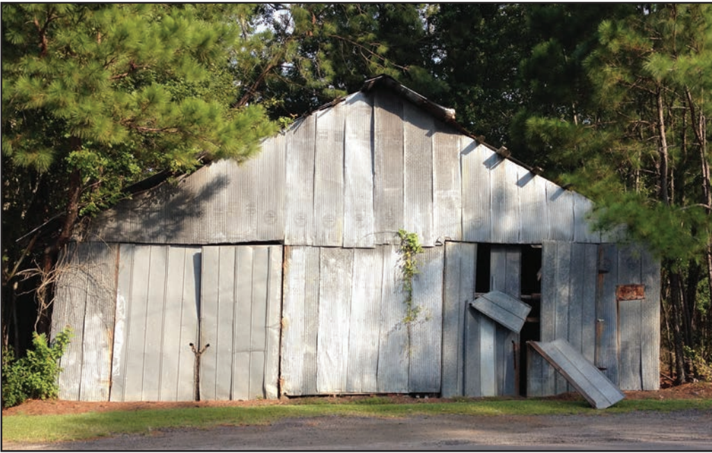
Plaintive beauty imbues this obsolete hay barn on Cooper Store Road across from the original Cooper family residence north of the State Road. Working farms feed families and fattened livestock for the Charleston butchers.
