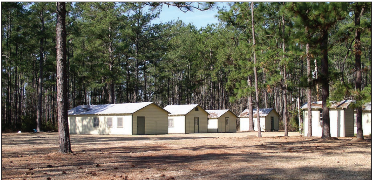
Below, "Duke's Camp," sitting 100 yards off the south side of the State Road, five miles beyond Cooper's Crossroads was a Prisoner of War detention center.
