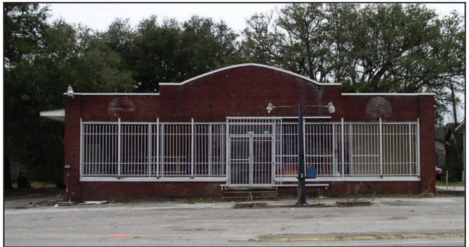
The Harvey Super Market is a rectangular frame structure with brick veneer façade and a curved parapet. White security bars span the front of the store when this image was taken in 2004. The large signs stating, “Harvey’s Super Market,” and “Texaco,” as well as two gas pumps were removed prior to this photograph. The image is among the collection of the author.
