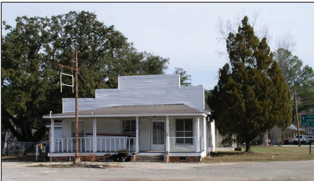
Cooper's Store , built in 1880 at the intersection of State Road (Highway 176) and Cooper Store Road. The store was a one-story frame building with a gable roof, screened by a parapet. A centered entrance was flanked by display windows and porch. The photograph taken in April 2003 shows the general store before it was razed in 2014. The photograph is among the author's collection.
