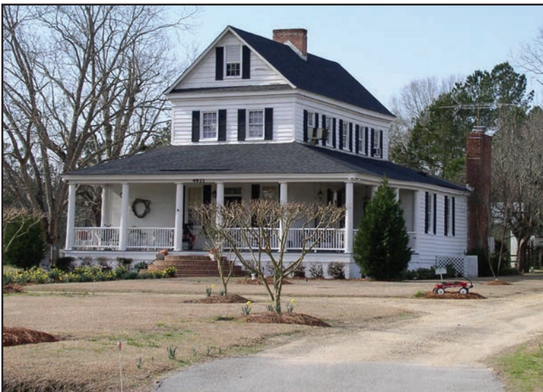
The photograph shows the Stephen Williams House of Sandridge, built in 1846 by the minister of the Springhill Methodist Church. The two-story frame dwelling features a front gable, central chimney and a one-story piazza across the front and part of one side of the structure. The house stands elegantly with cultured lawns, 19 miles west of Carnes Crossroads. The author took this photograph April 4, 2016. It is among the author’s collection.
